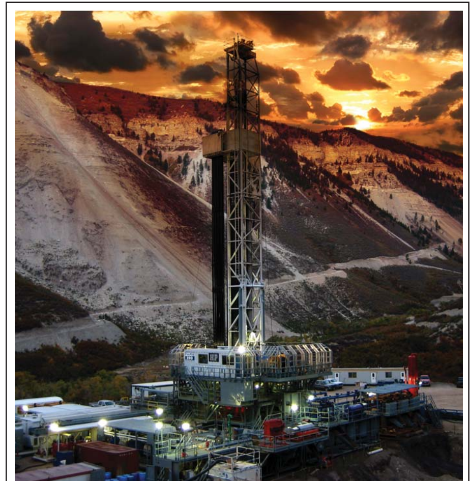
In response to increased demand, Helmerich & Payne International Drilling Co. implemented lean manufacturing principles to increase plant efficiencies and expand production of its newest-generation FlexRigs™, including this FlexRig4 unit.
